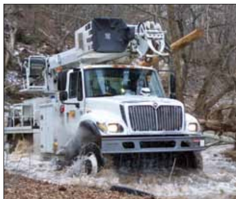
Bluestem linemen faced tough working conditions hindered by mud, stream crossings and rugged terrain.
