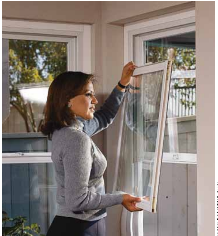
A single-hung fiberglass window sash frame can be removed for easy cleaning. Notice the weatherstripping on the edge of the sash.
